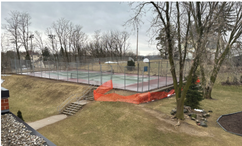
Tennis courts in need of repair
