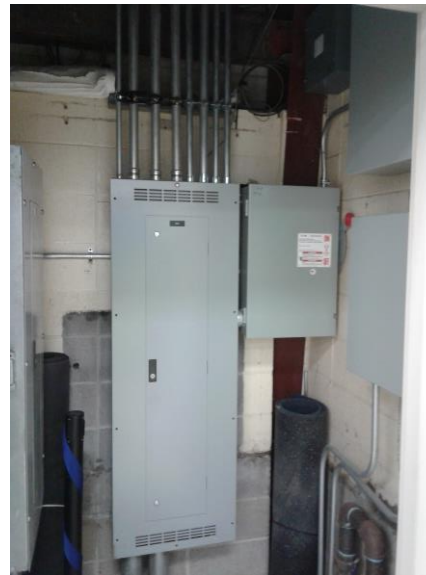
Extend fire alarm / panelboards
