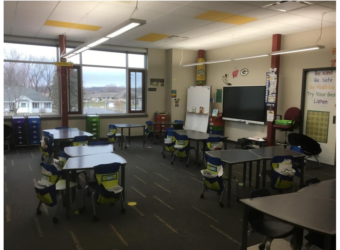
Replacement of fluorescent lights with LED
