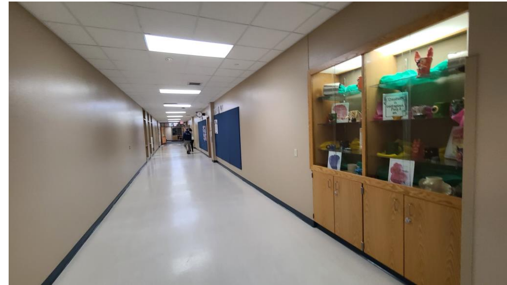
Ongoing replacement of fluorescent lights with LED; Fire alarm in need of maintenance/updating
